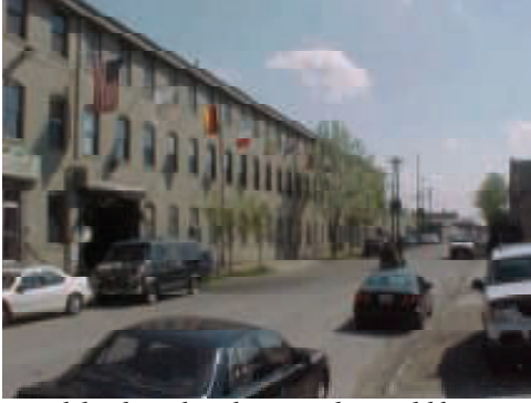
Consolidated Metal Products provides a model for potential adaptive re-use of former early 1900s industrial buildings.
