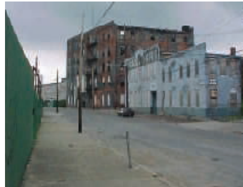
Blighted properties along Evans Street present significant safety issues and create a barrier between the existing Lower Price Hill Recreation Area and the residential population of the community.
