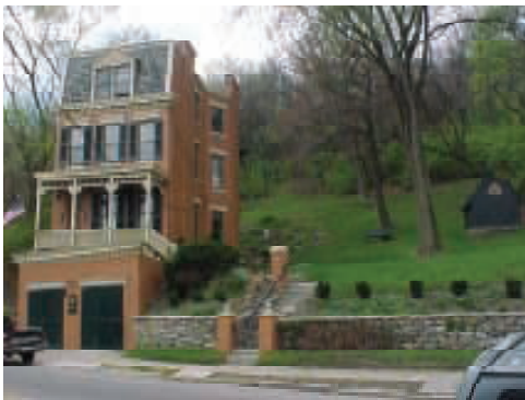
Many State Avenue residential properties have been rehabilitated despite their close proximity to Metropolitan Sewer District.
